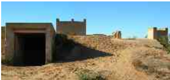
WWII radio communications bunker
