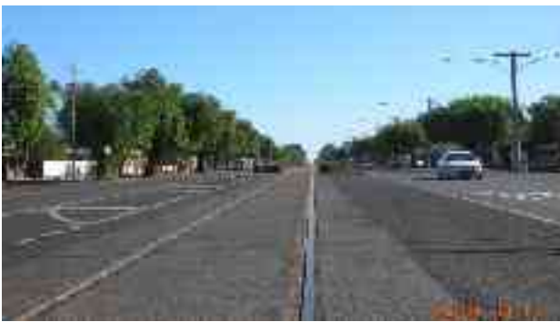
Railway track in centre of the main street
